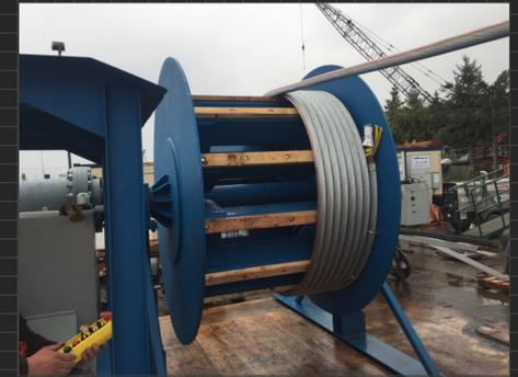
I-90 Floating Bridge Cable Replacement Powered Wire Spools, 2018, *Design Build*
